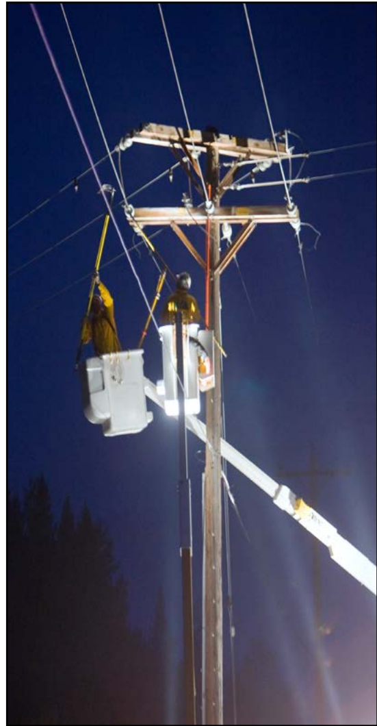
Figure 7.8. Utility companies begin repairing infrastructure and restoring service as soon as it is safe to enter the fire area.
