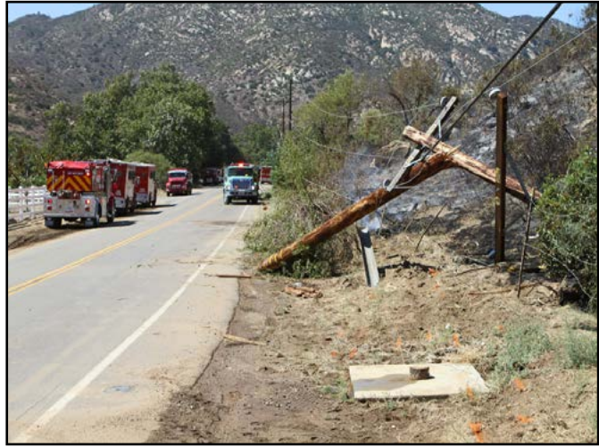
Figure 10.6. Firefighters should delay taking action when power lines are down until power company representatives advise that the power lines have been de-energized.
