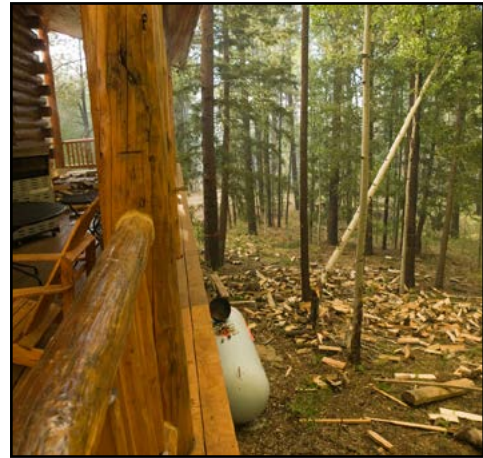
Figure 4.16. Evaluate hazards such as power lines and poles, and propane and other above ground fuel tanks, their clearance and their proximity to the structure. Photo courtesy of Kari Greer.
