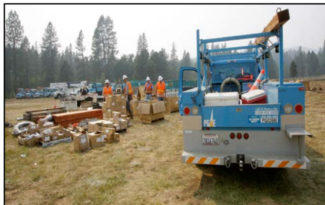
Figure 7.7. Utility companies can mobilize equipment and personnel similar to fire resource mobilization and are an essential cooperating agency for firefighter safety and the restoration of services.
