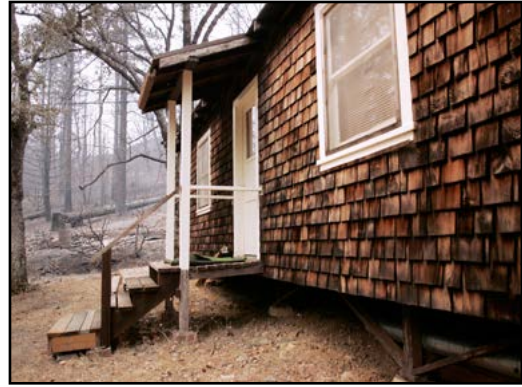
Figure 4.12. Flammable construction features such as shake siding or roofing, and ember traps such as open unprotected post and pier foundations are easily compromised when the fire impacts the structure.
