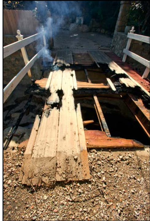
Figure 4.11. If bridges are constructed of flammable material, ensure they are secured with foam or gel pretreatment or post a firefighter at the bridge for exposure protection.
