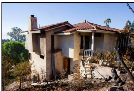
Figure 5.34. Tactical Patrol resources must focus on structures that sustained any degree of damage during fire front impact. These structures should be closely monitored throughout the operational period to avoid the possibility of re-ignition.
