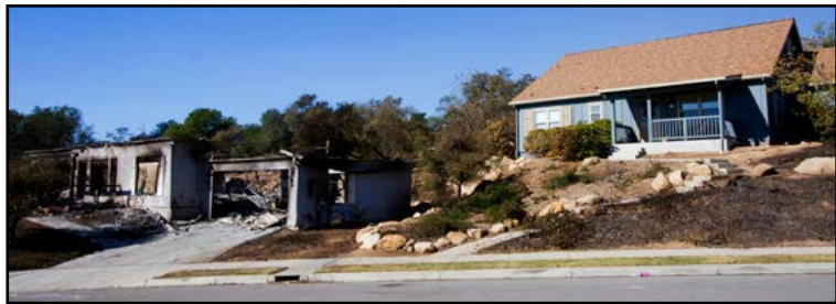
Figure 5.35. Resources must decide whether engaging a burning structure takes precedence over moving on to a threatened structure. Should resources protect the threatened structure and let the involved structure burn or take action on the burning structure and possibly lose both?
