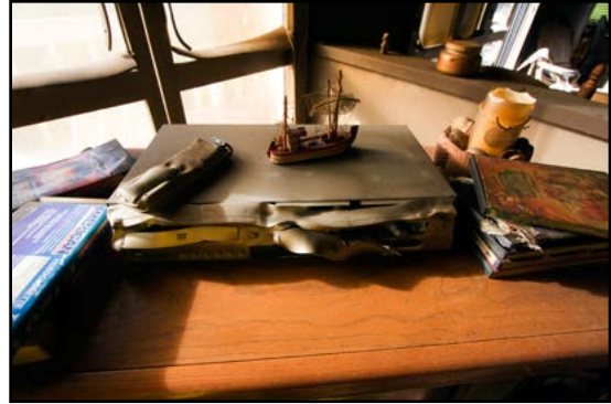
Figure 4.14. Melted window coverings and heat distorted video components are clear indicators of radiant heat intrusion through windows that could ignite interior construction components or furniture.
